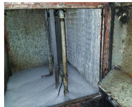
Figure 3: HRU washdown section showing clean coil.
